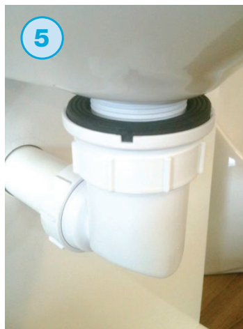
One-way valve goes in from above and threads into trap
