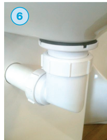
Adjust telescopic trap & tighten
